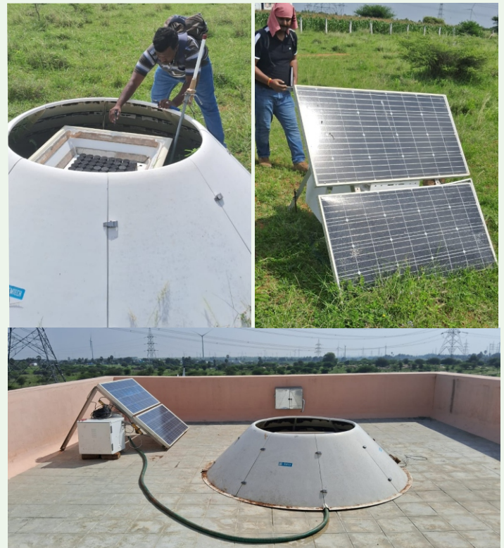
SoDAR rectification work at Kayathar
