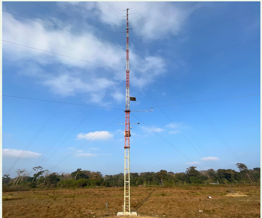
WMS Installed at Sigmundera
